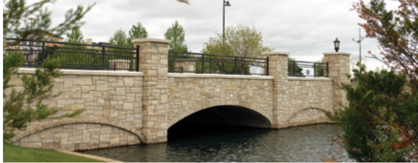
Speed Fab-Crete fabricated this bridge in Frisco. It has a single-cell arch with head walls and wing walls, and crosses a retaining pond and a 24-ft span with a stone finish and field set. (Photo Courtesy by Speed Fab-Crete.)
