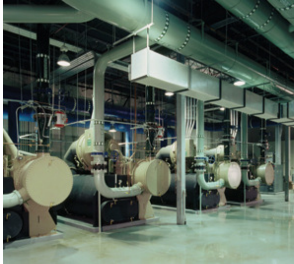
Brandt Engineering provided specialty contracting services at Dallas' Love Field Airport.
