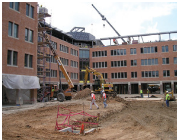
EMCOR's Gowan is installing HVAC and plumbing systems
